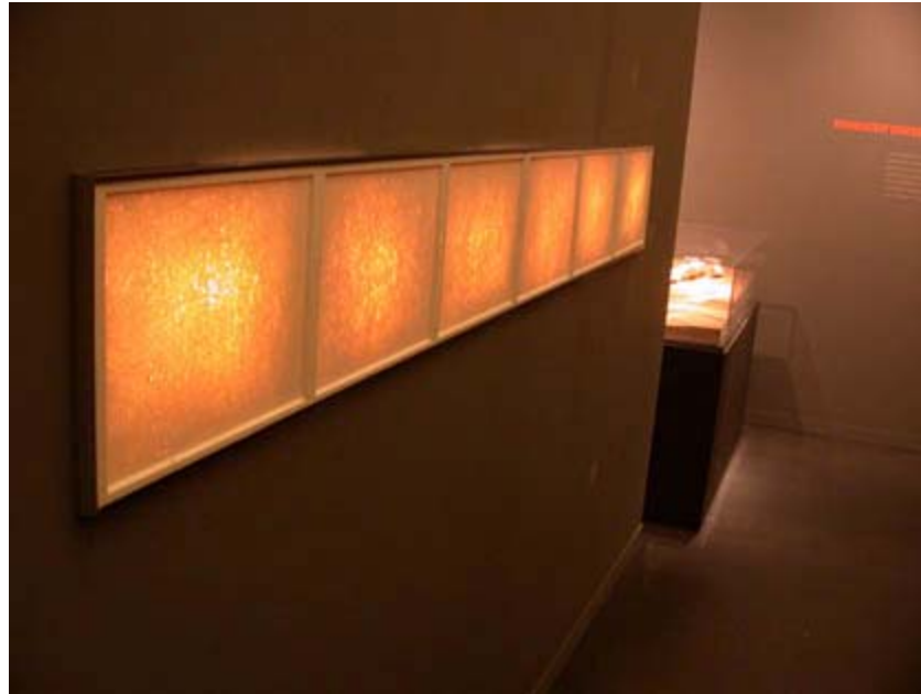
One of the translucent concrete panels in the Future gallery. Photo: Pure + Applied.
