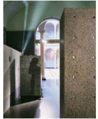
Future gallery w/ LiTraCon translucent concrete. Photo: Frank Oudeman.
